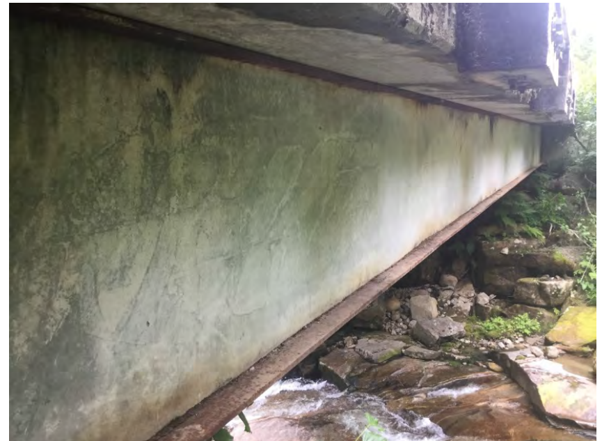
Typical Girder Condition
