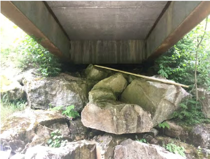
Left Bank Abutment
