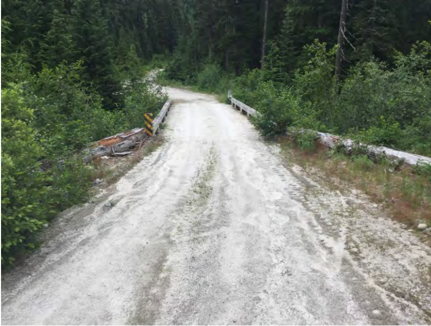
Right Approach Facing Bridge
