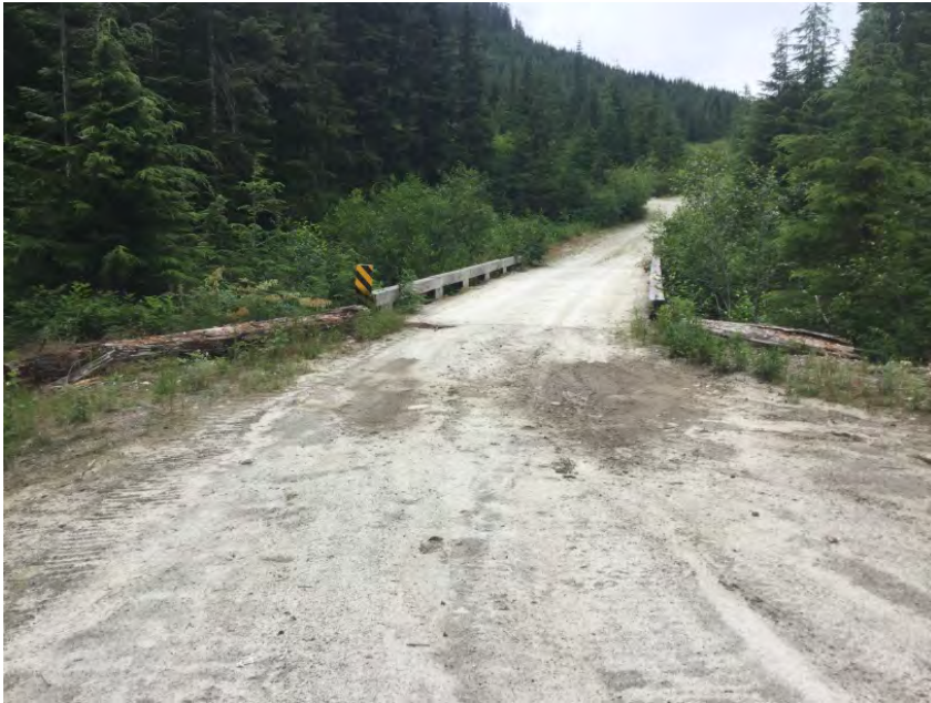
Left Approach Facing Bridge
