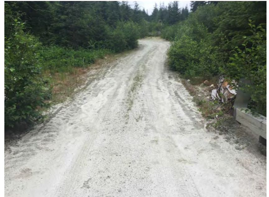
Right Approach Facing Away From Bridge
