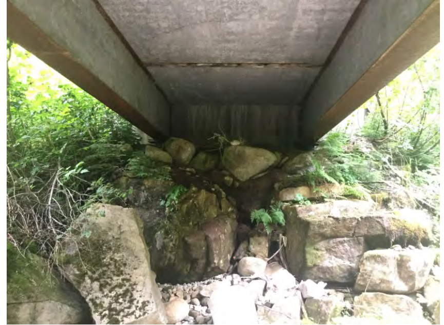
Right Bank Abutment
