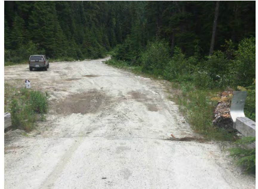
Left Approach Facing Away From Bridge
